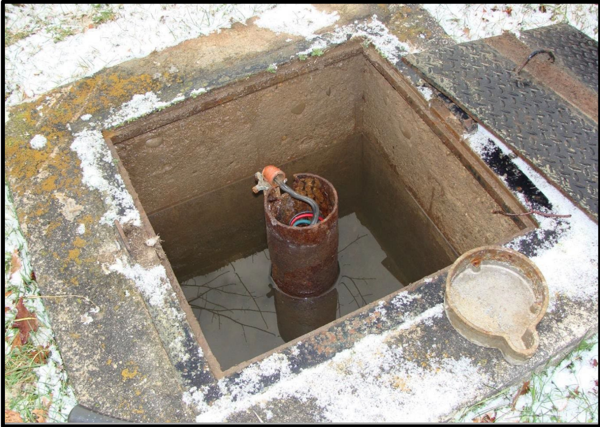
Figure 5: Potential Surface Water Contamination
