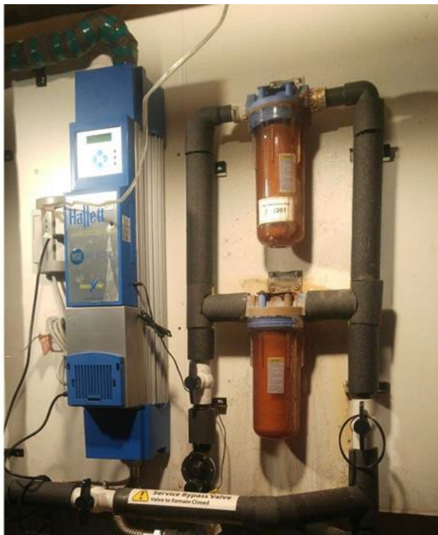
Figure 2: Ultraviolet Light System
