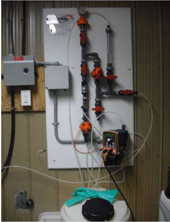
Figure 3: Chlorine Injector
