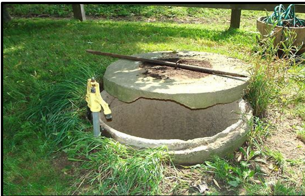
Figure 1: Damaged Lid and Casing
