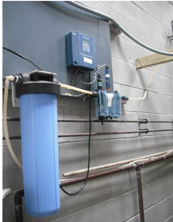
Figure 4: Chlorine and pH Monitoring System
