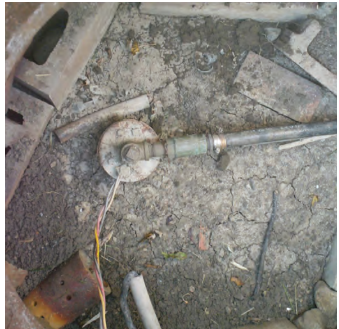
The soil is cracked, evidence that water has entered the well pit (not to be constructed this way anymore) and dried. One way to prevent this from happening is to upgrade the well by installing a pit-less adapter and extending the well casing at least 40 cm above the ground; and ensuring that construction/maintenance is conducted properly. New construction wells cannot be located in well pits. NEVER ENTER A PIT.
