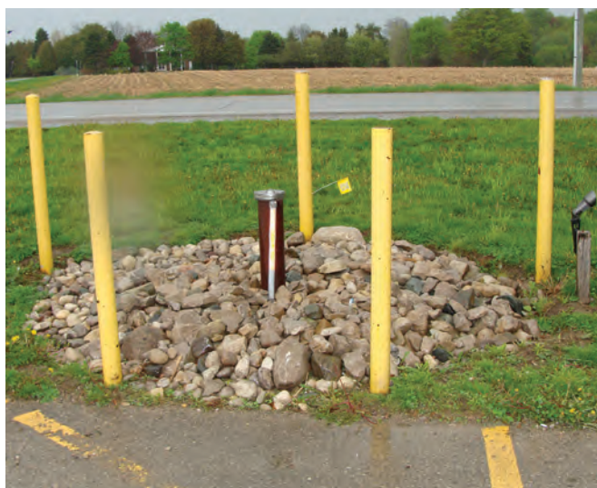
Wells located near the road or parking lots may be at risk of salt (sodium) and vehicle related contamination. Know what can get into your well and take measures to minimize the potential contamination and the risks.
