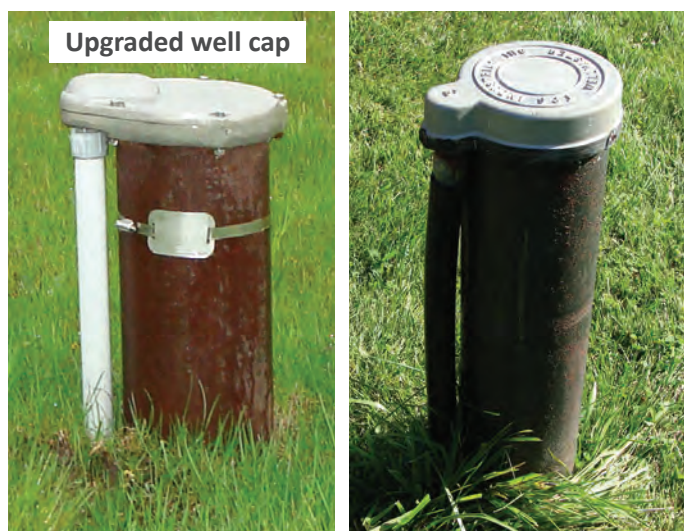
A properly constructed drilled well. The well cap should be upgraded to make the well more secure (pictured at left).
