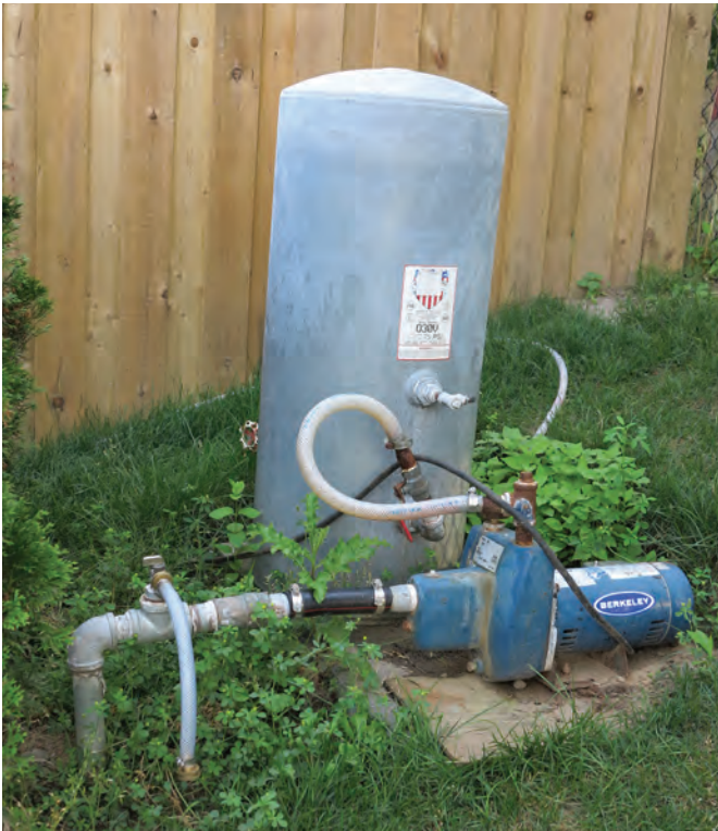
A well point (sand point) with a pump and pressure tank on the ground. These types of wells work in areas where the water table is high as they are not very deep. They are susceptible to surface contamination and changes in water table level. This well is used during the warmer months and winterized for colder months. Plumbing can also be installed below the frost line for year round use.
