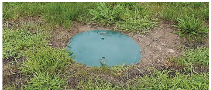
Septic systems can be a potential source of contamination.
